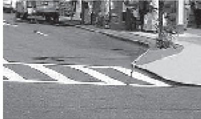
Curb extensions are sidewalks that project into traffic intersections to slow turning drivers and protect crossing pedestrians. They are also known as bulb-outs or neckdowns and extend the sidewalk or curb line out into the parking lane (one car length) which reduces the effective street width.
