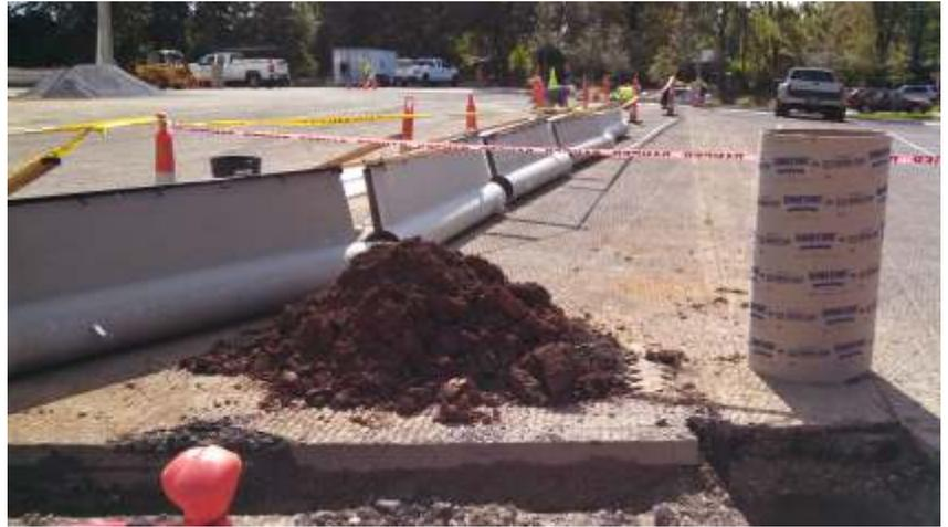
For sandy or less firm soil the bars will have to be driven deeper to resist flotation forces.
