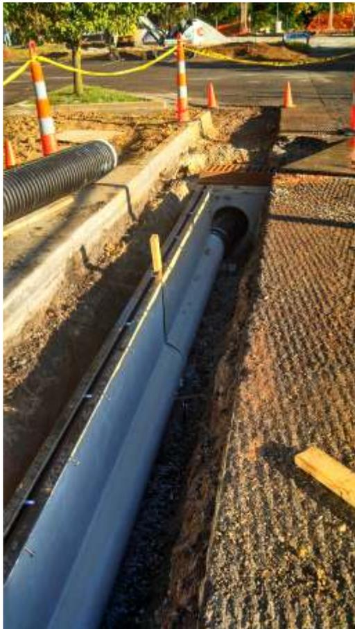
beside the trench and use tie wire to pull trench in line with the string and to ensure that the trench will not move during the concrete placement. Deeper slot drain throats are more likely to need additional bars to align the trench sections.
