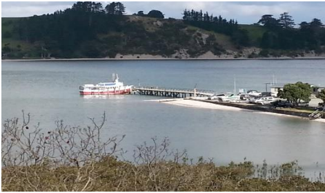
QP2 at Pahi Wharf
