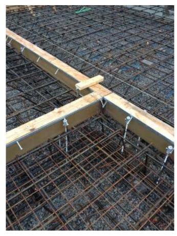
string. This will ensure that the trench will not move during placement. Deeper trench sections are more likely to move and need additional bars to align the trench sections.
