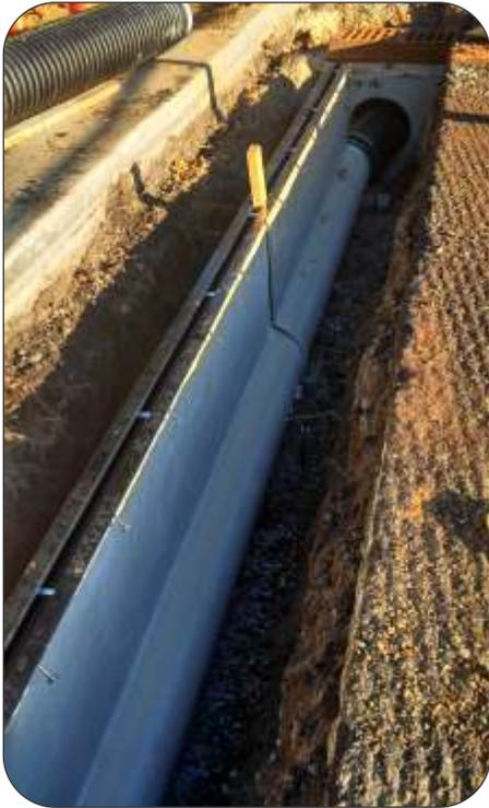
The Dura-Trench Slot drain comes standard with built in slope. Non-sloping drainage products just don't make sense. Typical slopes are 0.5% or 1% and really get things moving! The ultra smooth interior flow line not only moves considerably more water than similar products, but also passes debris and solids easier due to increased flow velocities.
