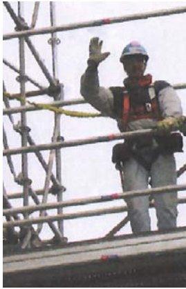
Tim Trask on scaffolding at Lepreau
